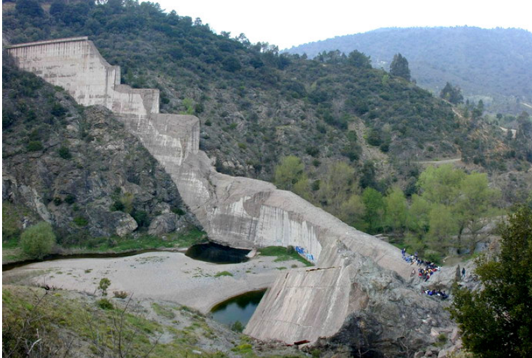
Figure 1: Remains of the Malpasset Dam as seen today. Photograph by Mark Diederichs, 2003.
